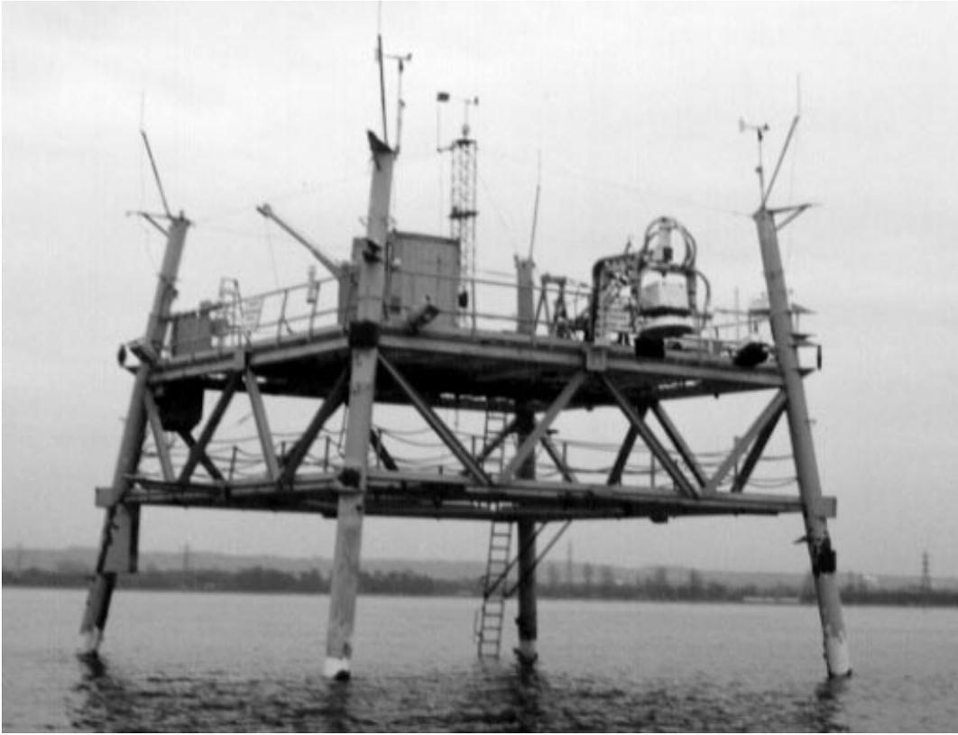
Figure 2.3: The Canada Centre for Inland Waters (CCIW) WAVES research platform. YSCAT is the crane-like structure on the upper deck. Also visible are the two anemometers on the support legs and the bivan anemometer on the tower in the center of the platform.
