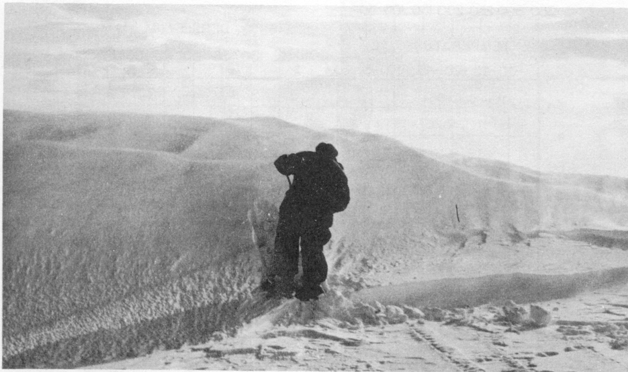
Figure 7g. Snow drift formed between 0200 and 1400 at station 00-20 on 12 June 1954. The tracks which go under the drift were made 12 hr before this photo was taken.
